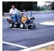
Parking Lot Striping
